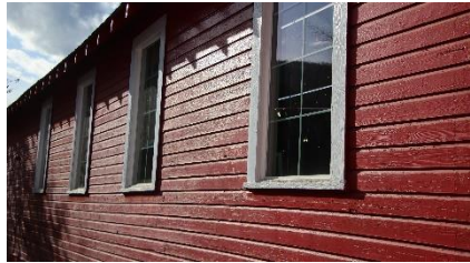
Windows on south elevation
